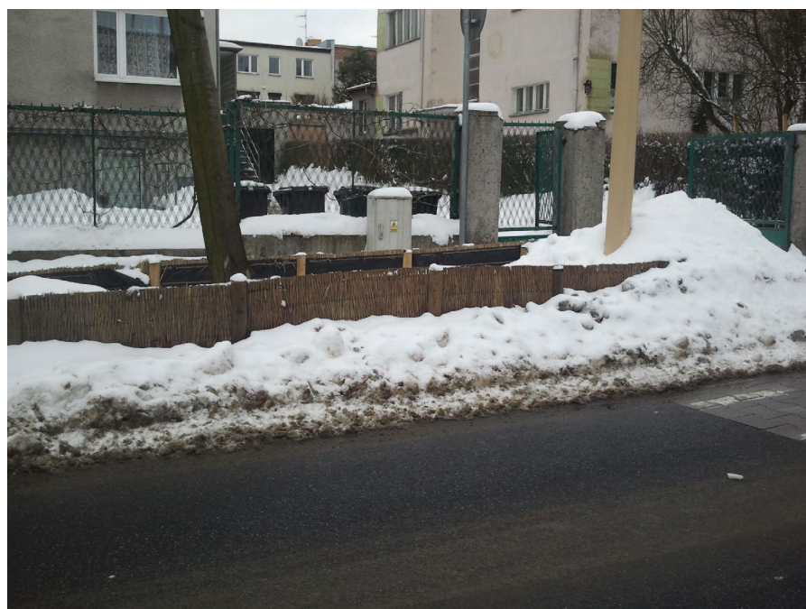
Fig. 6. Snow piled inside barrier fences put up to protect roadside vegetation from the adverse effects of road salt, Poznan (photo by J. Dąbrowska)
