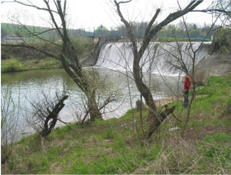
Figure 2. Uswicza River in Brzesko. The 5.3 m high weir built in 1913 was not equipped with any device for animal migration until 2020 (photo by M. Klich, 20.04.2004).
