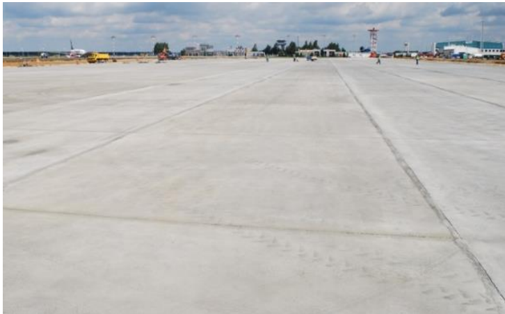
Fig. 1. Rigid pavement of cement concrete
