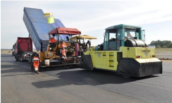
Fig. 5. Paving the mineral-asphalt mixture (paving the asphalt concrete)
