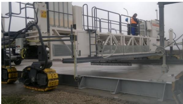
Fig. 4. Texturing of the surface from cement concrete
