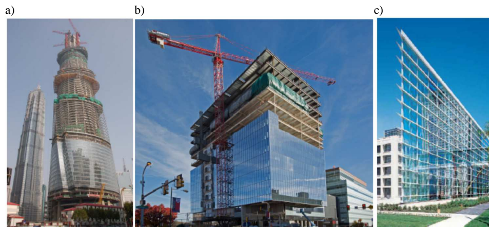
Fig. 6. Construction of curtain walls, architectural systems broadly utilising the principles of modular design; manufacture and on-site assembly: a) Shanghai Tower Curtain Wall (China), b) Science Research Centre, Wausau (Pennsylvania/US), c) Stick System curtain wall Reliance™ manufactured by Oldcastle
