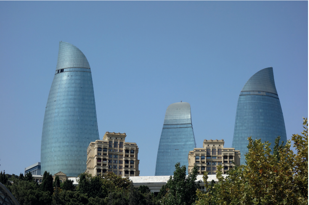
Fig. 12-43. Flame Towers dominating the skyline of Baku in a view from the interior of urban tissue and in the perspective of the horizon, design by HOK. Photo by E. Kaczmarzka
