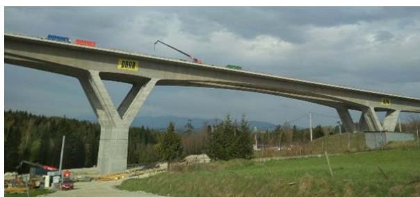
Fig. 6. A fragment of the longest flyover on the Skomielna Biała–Chabówka section III (992 m long; largest: span the span 140 m, height of the support together with the supporting structure 49.4 m) [source: 12]
