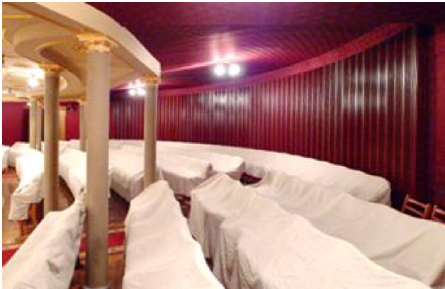
Fig. 17. The underbalcony space in the Lviv Opera House after mounting the sound diffusers.
