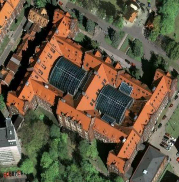
Fig. 18. Glazing roofs over Gdańsk University of Technology's main building courtyards (Google maps, 2015).
