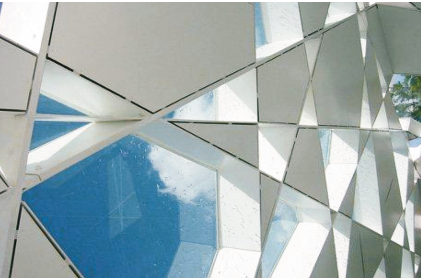
Fig. 6. Serpentine Gallery Pavilion 2002, London - Next steps in generating the construction system; source: openbuildings.com
