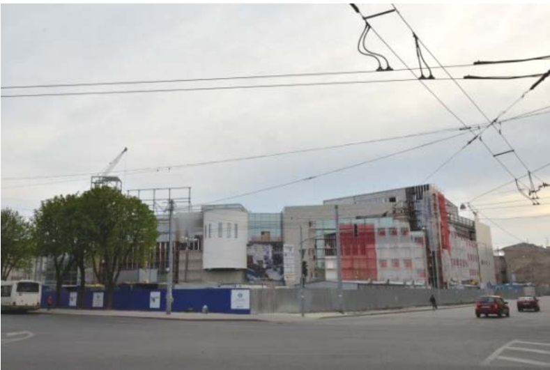
Fig. 3. Former factory JSC "Gas Equipment". Construction of the new shopping centre Forum Lviv. Source: photo Y. Senkovska
