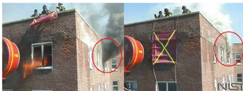
Figure 17. Use of wind protection curtains
