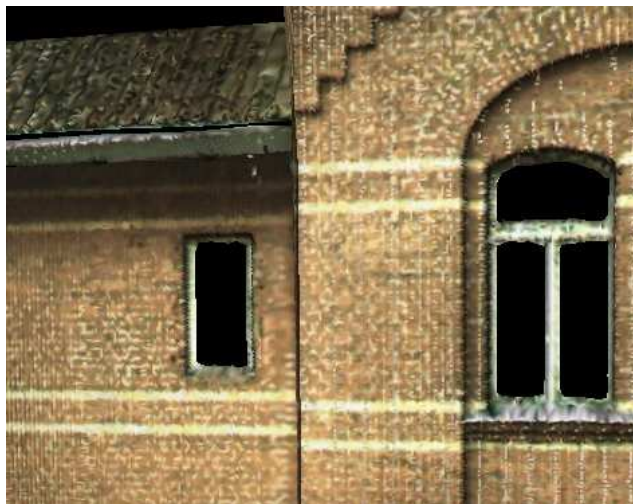
Fig. 3. The same fragment of the facade (see Figure 2) modelled using TIN grid (source: own study)
