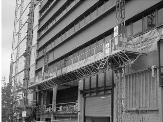
Figure 1. A HEK (USA) climbing platform, manufactured to eliminate difficulties with scaffold footing, removable guardrails, and variable cross bracing.
