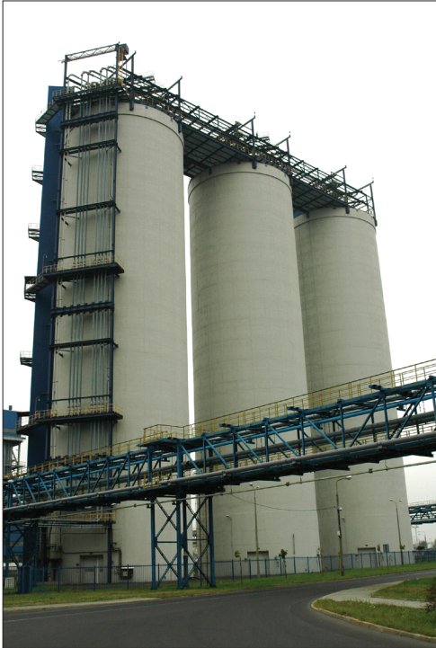
Fig. 1. Fly ash silos in a power plant (structure)
