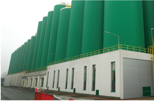
Fig. 3. Fermentation tanks (parts of a process installation) based on a production building in a brewery
