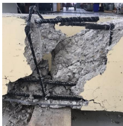
Fig. 5. Detail of destruction of beam with BFRP reinforcement
