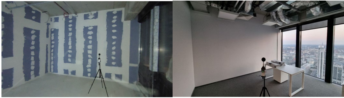
Figure 3. View of the wall in the receiving room. From left: stage 1 and stage 2.
