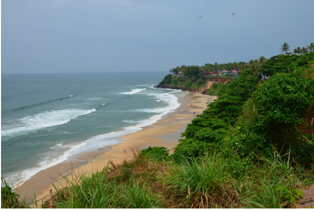
Fig. 3. Cliff coast at Varkala. The development of cliff is conditioned by subterranean flow of water, resulting in removal of underlying clay materials and accelerated retreat of the cliff face
