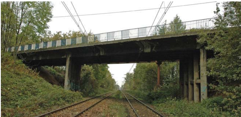
Fig. 1. South side view of the viaduct
