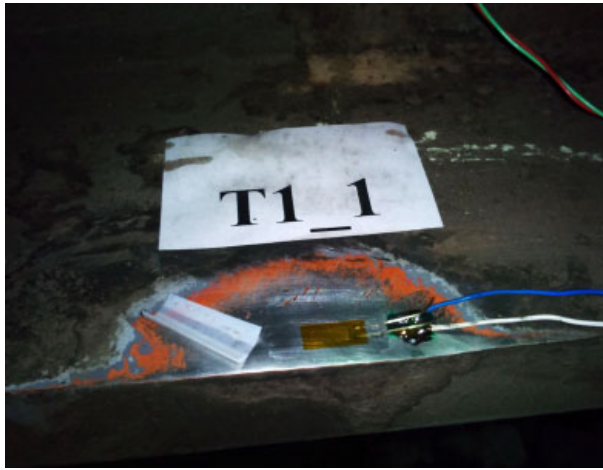
Fig. 4. Strain sensor T1_1 attached to the lower flange of the beam 1
