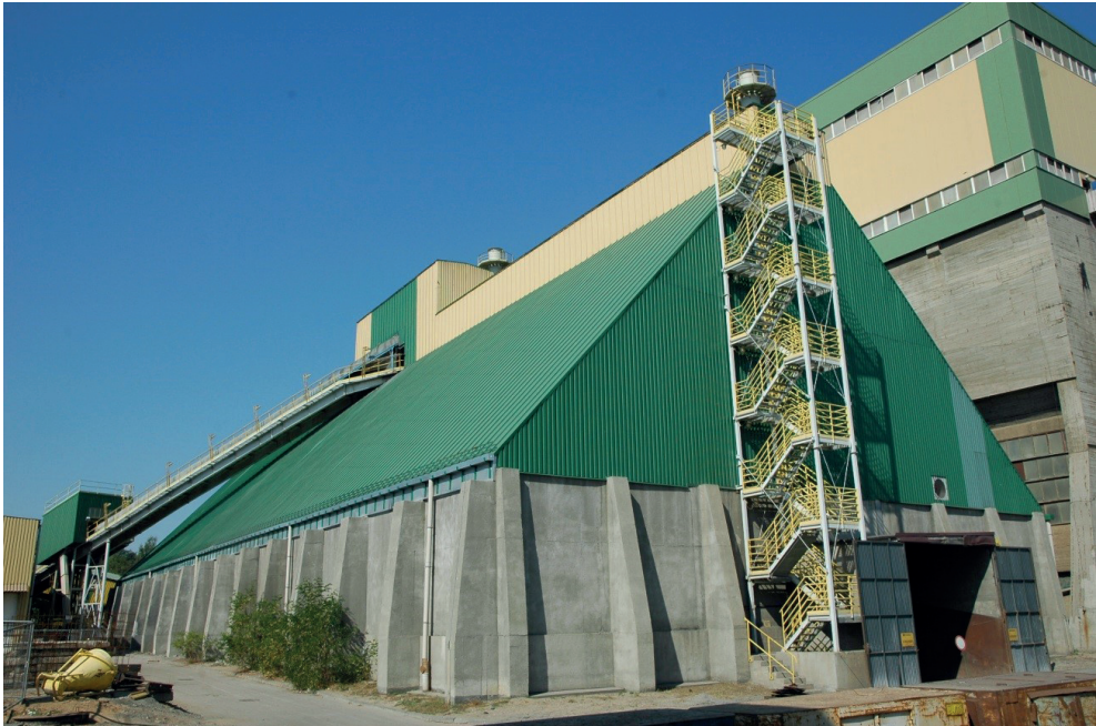
Fig. 1. Copper ore warehouse at the industrial plant – a building
