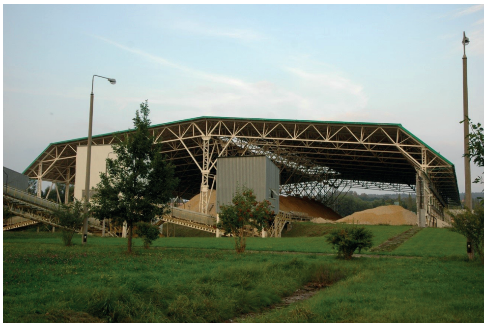
Fig. 2. Limestone storage site at the industrial plant – a structure
