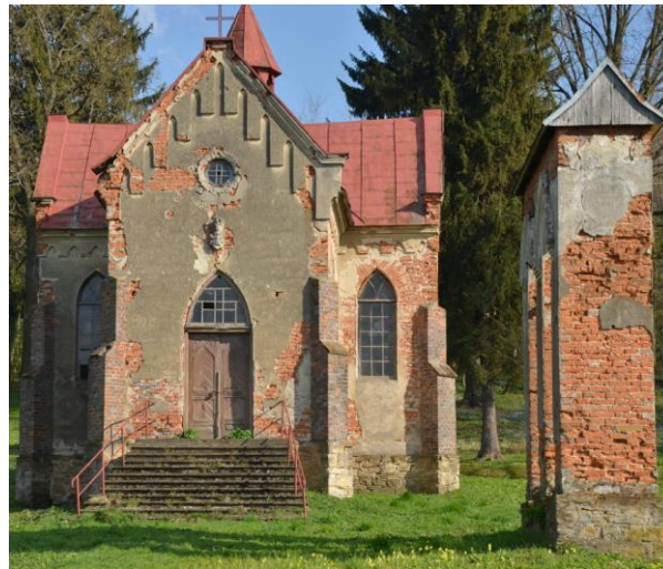
Figure 1. An example of a historic building in which the historic fabric has been destroyed as a result of the abandonment of modernization efforts (own source).
