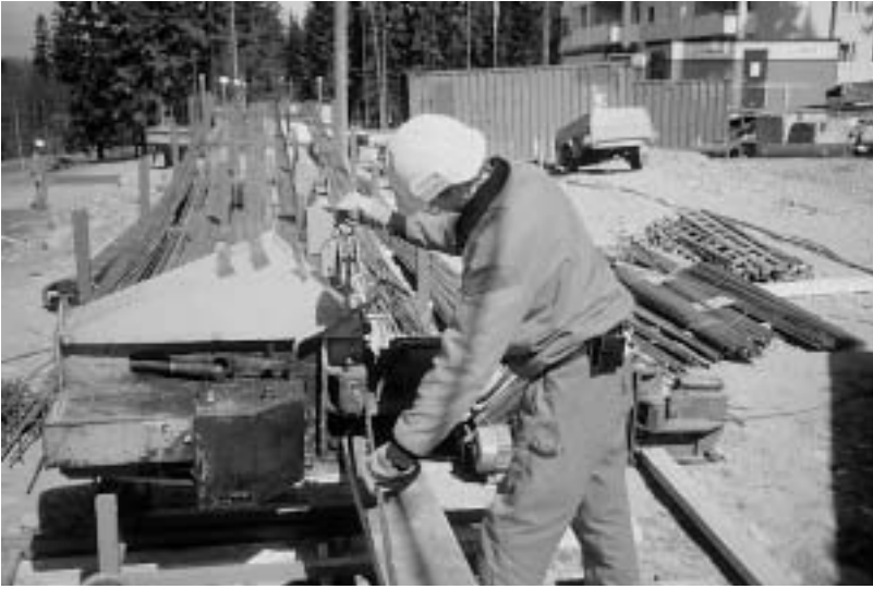
Figure 4. Moving and cutting concrete reinforcement rods with the new method.
