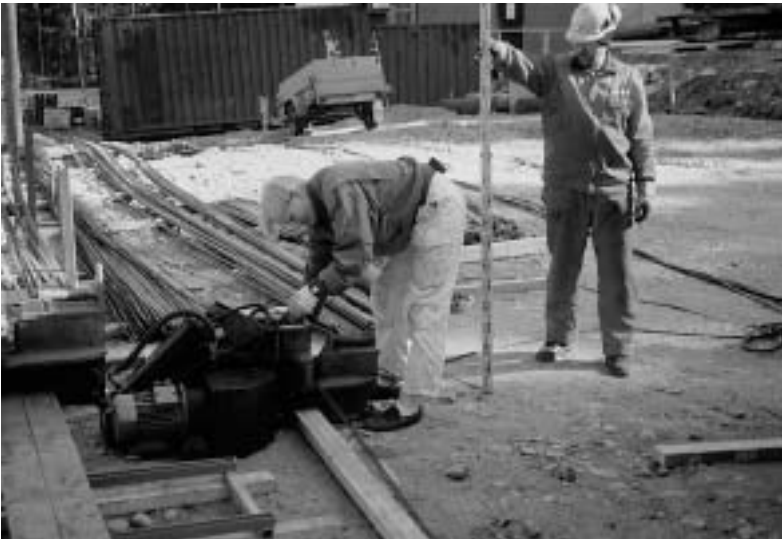
Figure 3. Moving and cutting concrete reinforcement rods with the old method.
