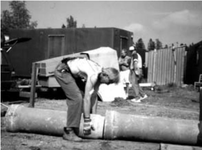
Figure 7. Fitting drain pipes with the old method.
