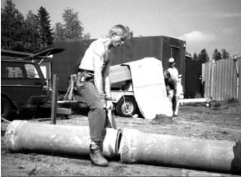
Figure 8. Fitting drain pipes with the new method.
