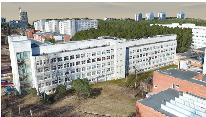
Fig. 4. Developed photogrammetry model of the building (source: own study)
