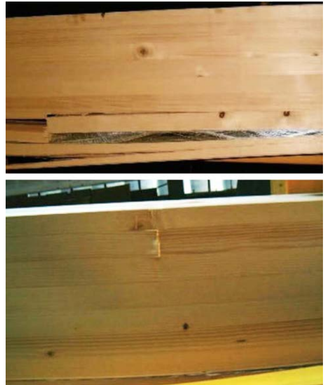
Fig. 5. Examples of failure of reinforced beams during Brol's tests [2]
