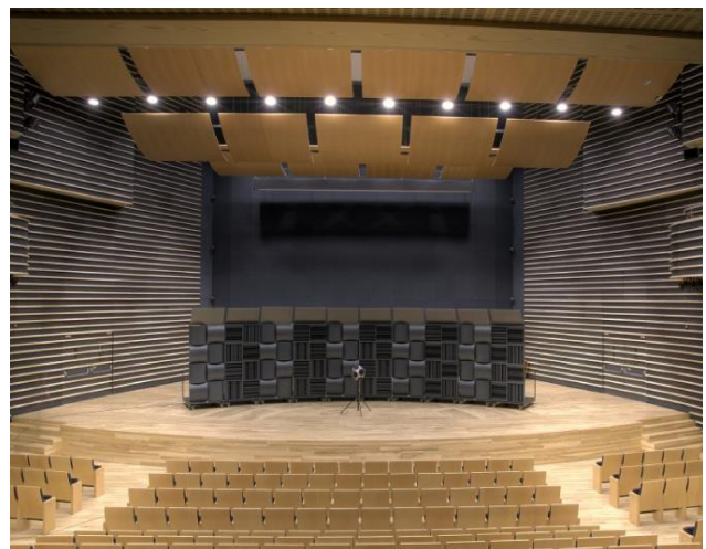
Fig. 1. The reflective panels which provide appropriate transferring of sound waves' reflection, Feliks Nowowiejski Warmia and Mazury Philharmonic, Olsztyn (photo by Piotr Pękala).
