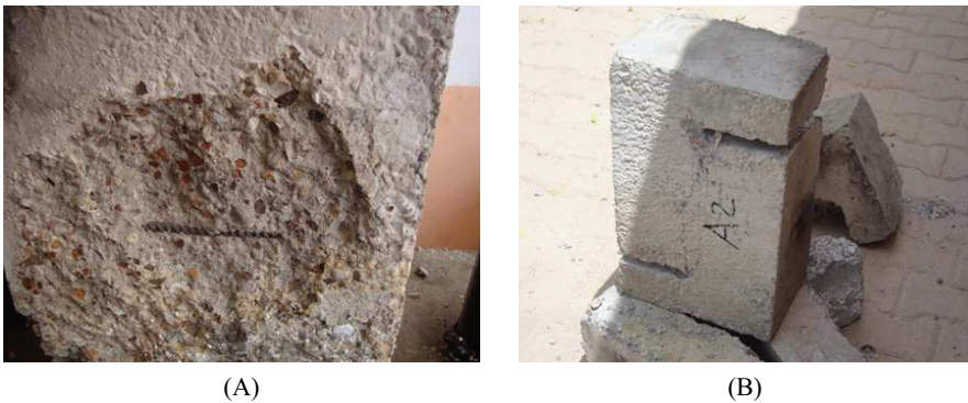
Fig. 5. Effects of direct fire (A) after three hours. (B) Second surface which was not exposed to fire.
