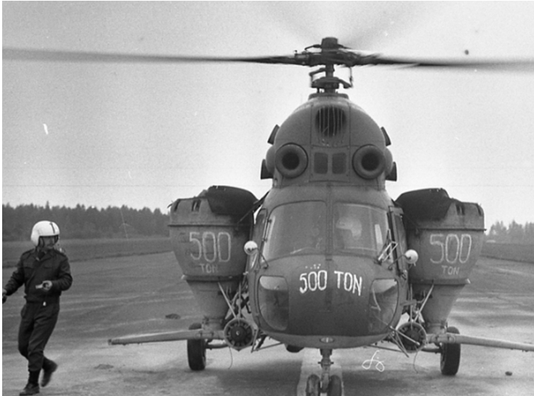
Fig. 4. Agricultural equipment of a military Mi-2 helicopter. Jan Piotr Urbaniak's file.
