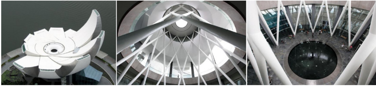
Fig. 14. The dish-like roof form collects rainwater; source: https://arthescience.com/blog/2016/01/19/spaces-artscience-museum/ , https://archello.com/project/the-artscience-museum-at-marina-bay-sands
