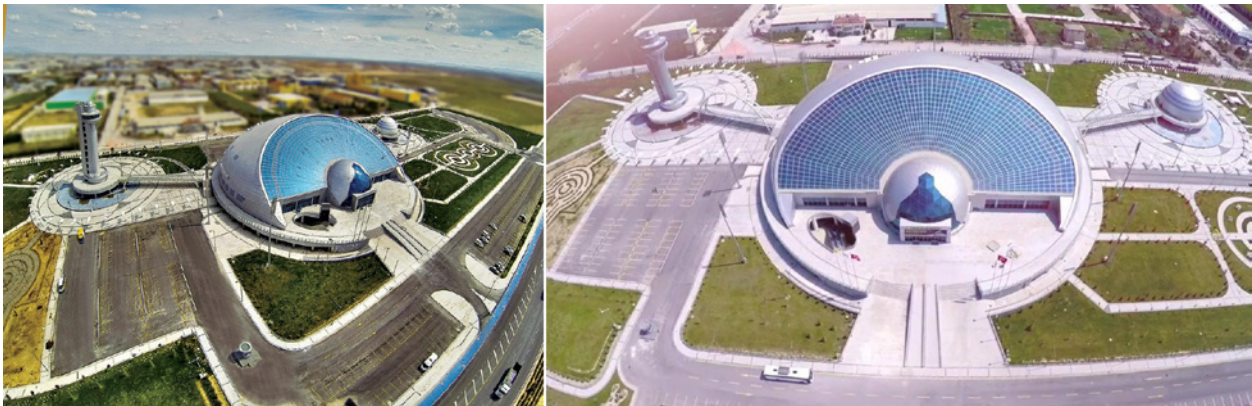
Fig. 5. Location of Konya Science Center, 2014, general view, 2014; source: www.konya.bel.tr/haberbasin.php?haberID=4111&hDurum=FOTO
