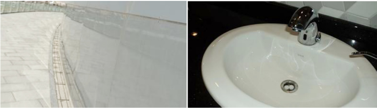
Fig. 8. Rainwater channel and high efficiency sensor battery; photo by the author
