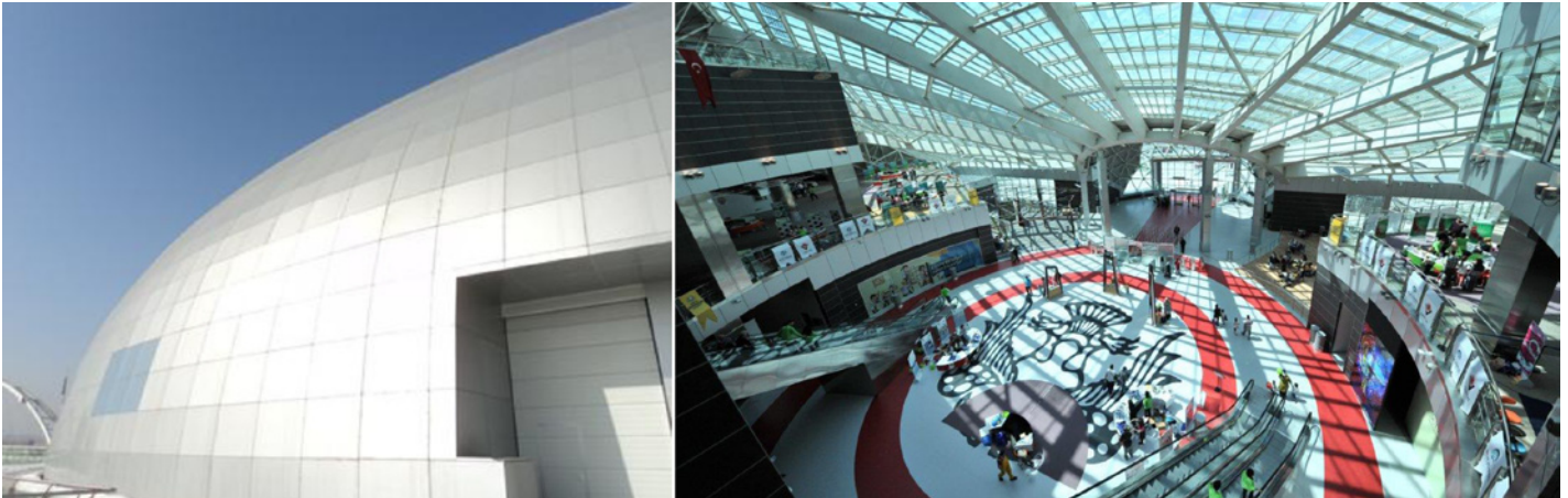
Fig. 9. Facade material that reflects the sun's rays by 90 % and using steel materials; source: photo by the author; http://ogm.meb.gov.tr/www/konya-bilim-merkezinde-fen-liseleri-matematik-zumre-baskanlarina-yonelik-uygulamali-egitim-programlari-basliyor/icerik/775
