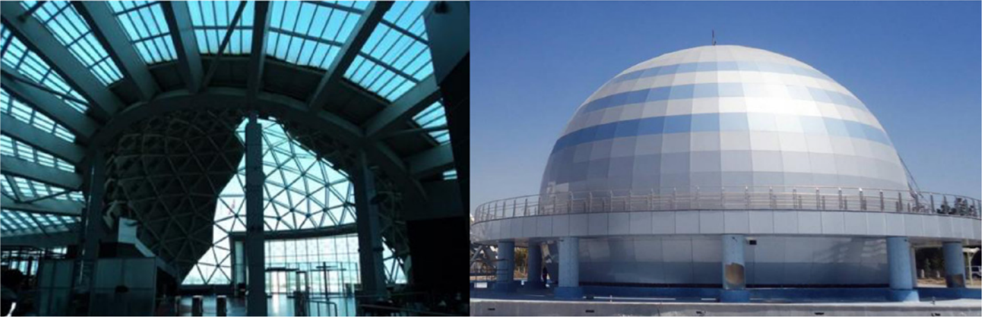
Fig. 6. Konya Science Center steel mesh shell system and geodetic shell; source: www.yenihaberden.com/bilim-merkezi-konyanin-markalarindan-biri-olacak-31967h.htm
