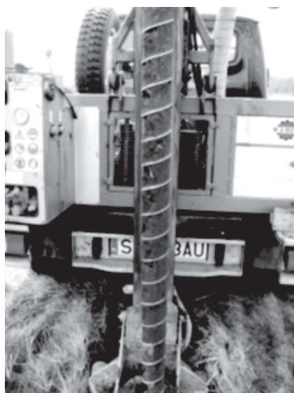
Fig. 4. The auger filled with an ash-slag mix
