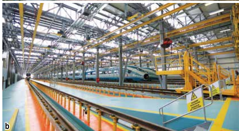
Ankara high speed maintenance center: a) external view, b) internal view
