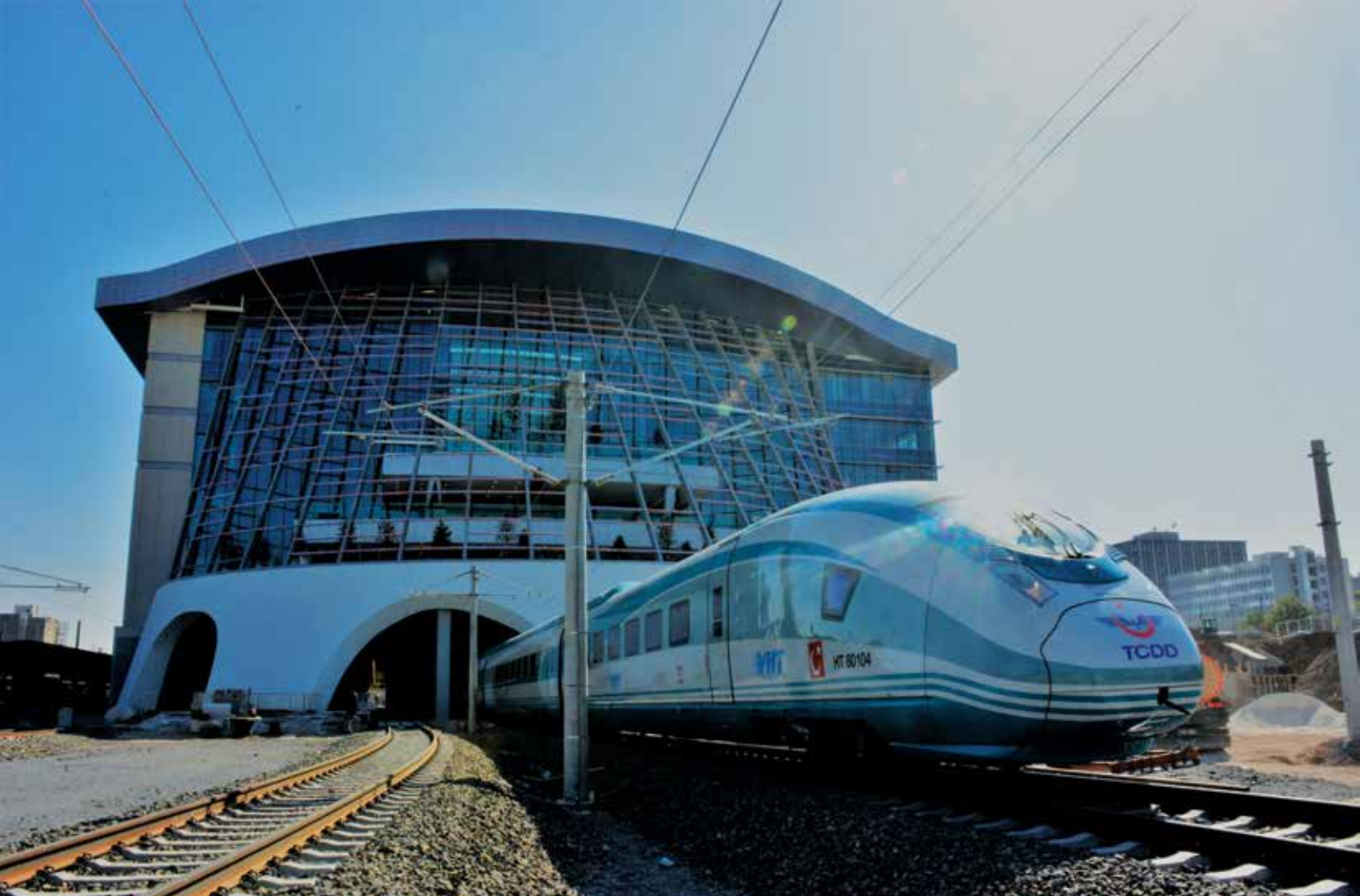
Overpass on High Speed Railway Ankara-Sivas (km 449)
