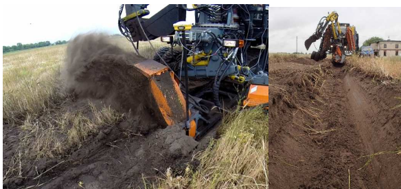
Fig. 12. Performing the drainage groove by scraping plough-share with a rotary desilting machine
