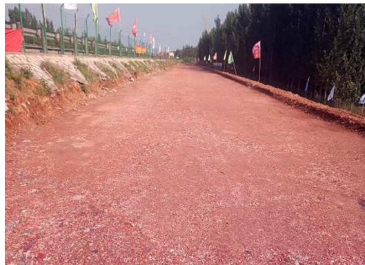
Fig. 14. Coal gangue roadbed
