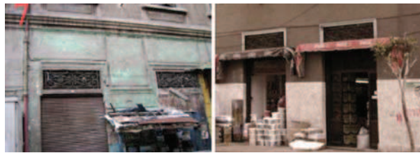
Fig. 13. Photos representing the store front of the building (Source: the author, 2010)
