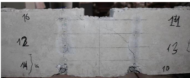
Fig. 9. Display of formed cracks in beams BD.80-0
