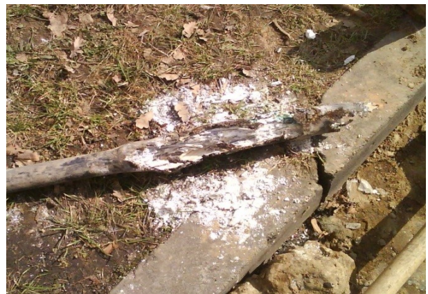
Fig. 10. A view of the consequences of the oxidation process
