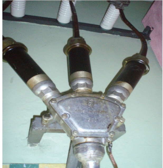
Fig. 2. View of a cable head of the 3GOw type
