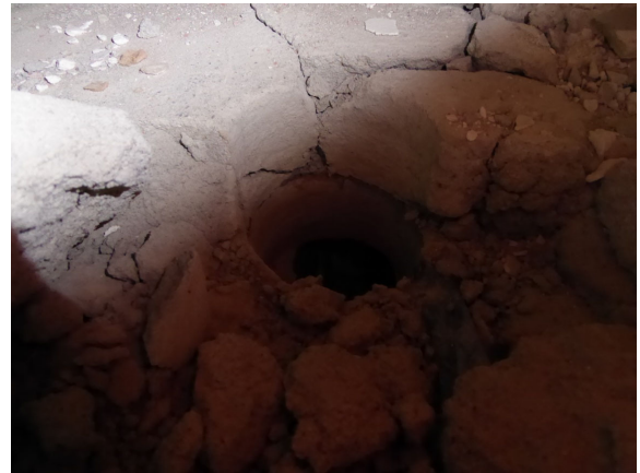
Fig. 3. View on floor layers during scheduled demolition work
