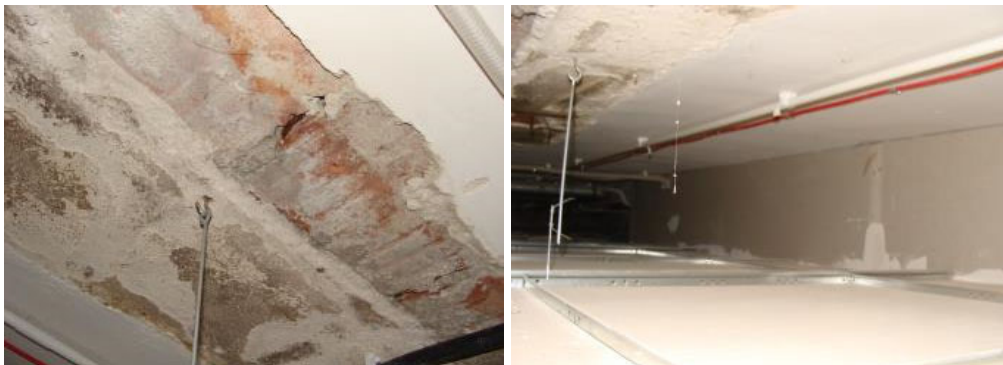
Fig. 2. View at the construction of Ackerman ceiling from the bottom
