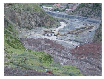
Fig. 2. General view of the hydrotehenical structure of Kazbegi HPP being constructed in the Gorge of river Tergi as a result of the mudflow formation (17.05.2014)
