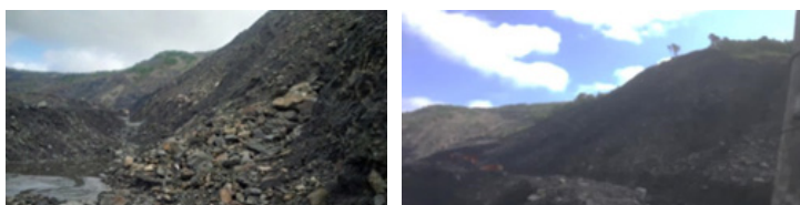
Fig. 1. The waste dump site at Mong Duong-Coc Sau mine: a. Foot of the waste dump site, b. The slope of waste dump site
