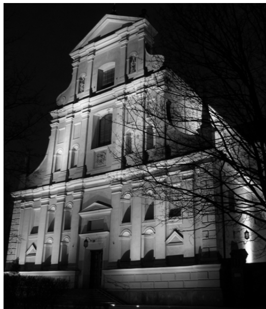
Fig. 9. Execution of the St. Joseph church illumination
