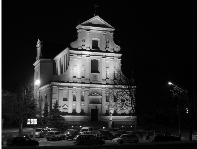
Fig. 10. Execution of the St. Joseph church illumination
