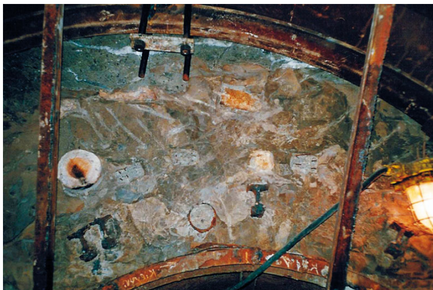
Photo 1. Sealing plug at the end of transverse Mina
