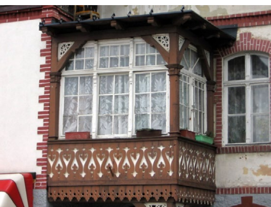
Fig. 23. Karpacz, veranda combining wood and wall structure (photo A. Borcz)
