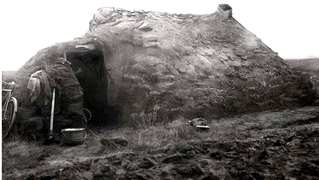
Fig. 8. Dutch settlement in the rural. Wooden residential buildings on stilts pitched on the island of Marken (province of North Holland, the end of the nineteenth century) – at the top and property of turf and peat blocks in Emmen (province of Drenthe, 1922) – at the bottom. Source: [27] – in advance, [13] – bottom
