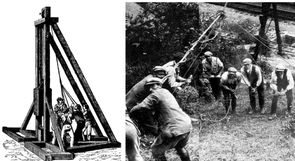
Fig. 12. Manual driving of the pile of wood by a group of men (8–12). Source: [16] – left, [19] – right
