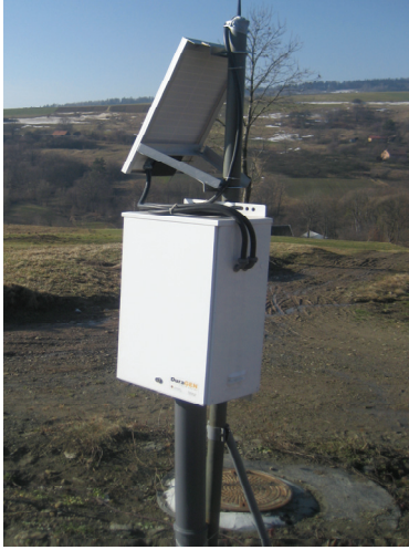
Fig. 6. Continuous 3D inclinometer on-line station
