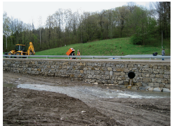
Fig. 13. Stabilization works at Sekowa landslide
