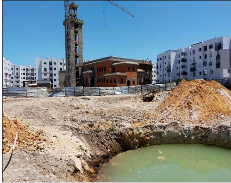
Fig. 1. In-ground basin adjoining
