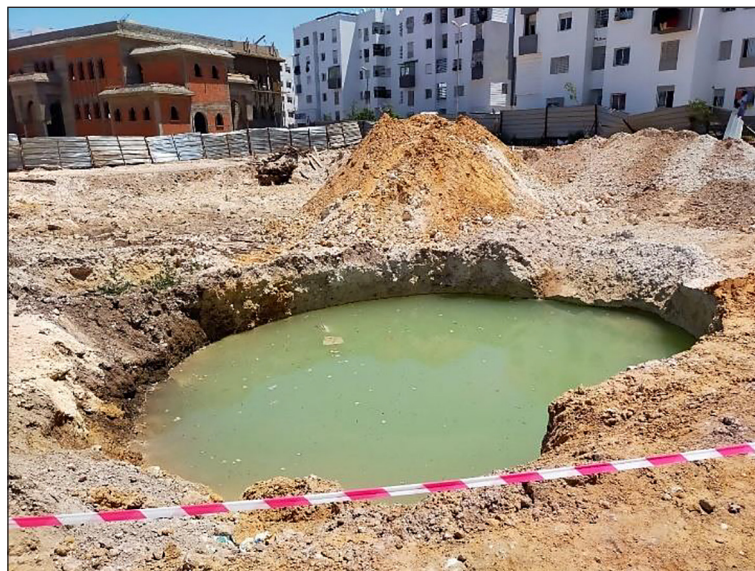
Fig. 2. Underground basin site
