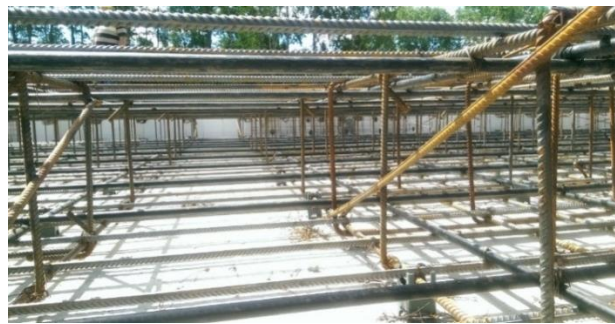
Figure 3.3. Top slab reinforcement
