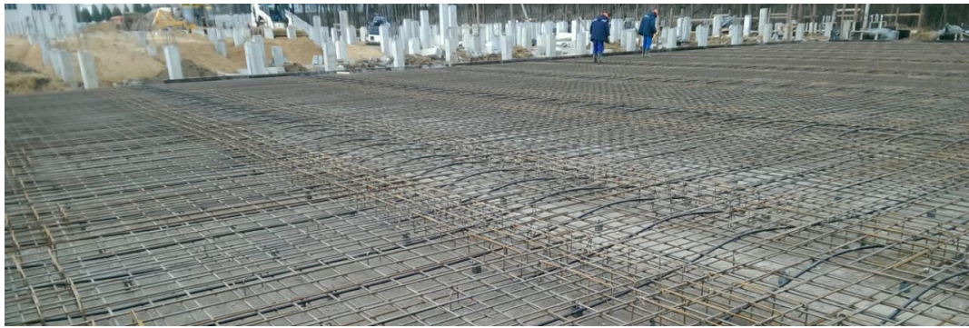
Figure 3.2. Tracing of the tendons
