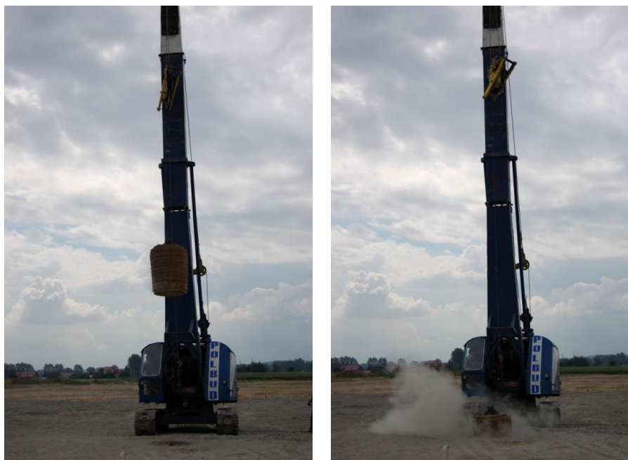
Fig. 5. Dynamic soil compaction (A2 motorway, Kolo-Dąbnie section)
