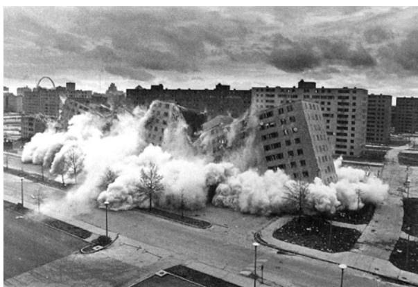
Il. 8. The spectacular moment of the demolition of the Pruitt-Igoe development in 1972, which was built in St. Louis in 1955. Source: Roger Trancik, Finding Lost Space, Theories of Urban Design , New York 1986
