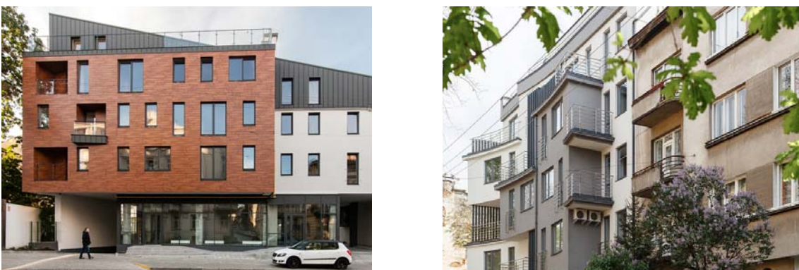
Fig. 2. New infill building in historical area of Lviv), architectural workshop „Zelemín”: a - Lviv, Pekarska str. 30 (2017); b - Lviv, Hlyboka str. 7 (2013).
