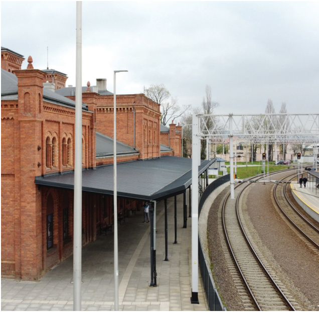
Fig. 11. Real space, a traditionally understood railway station building (source – author)
