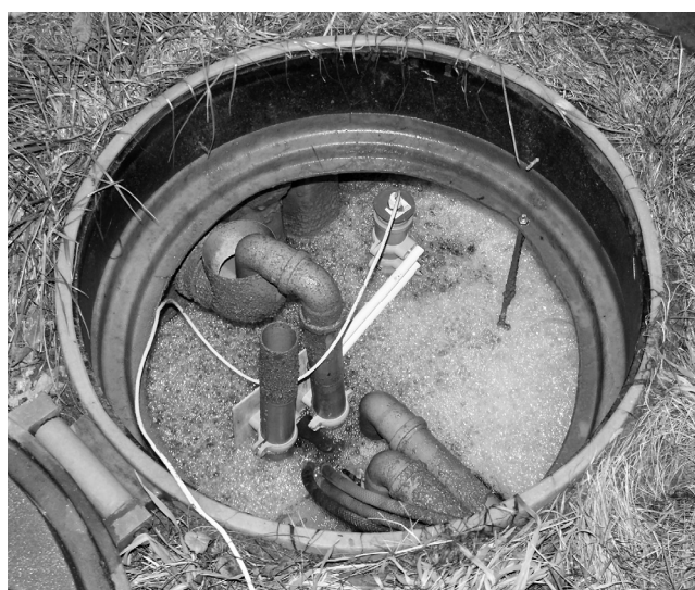
Rys. 1. Reaktor oczyszczalni Fig. 1. The reactor of the sewage treatment plant
