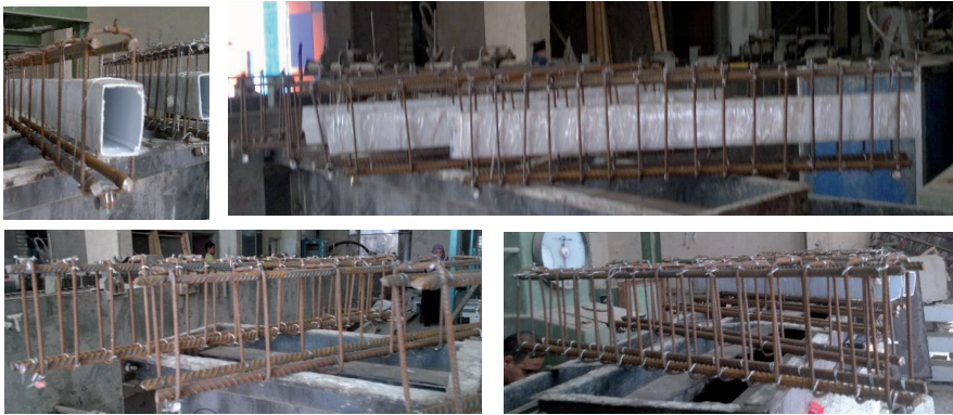
Fig. 2. Photo Showing Reinforcing Bars with Plastic Box for Specimen
